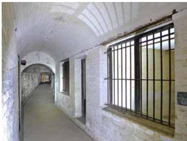
Rooke Battery: part of the underground works. The tunnel to Hayne's Cave Battery is beyond the arch; the magazines lie to the left, at a deeper level
